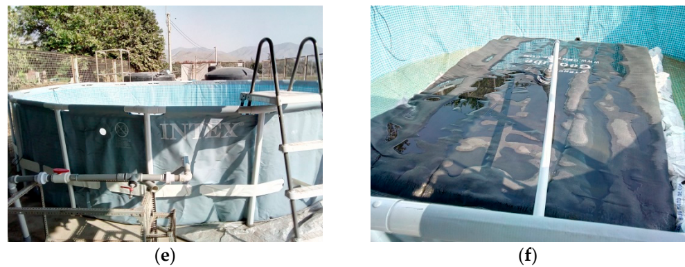
Figure 3. (a) Aerial image of the experimental area at INIA. The color of the reservoir water is an indicator of the concentration of algae. Water treatment plant images: (b) pumping system of the Rímac River water reservoir; (c) dosing pumps, (d) serpentine mixer, (e) treated water reservoir, (f) geotube.
